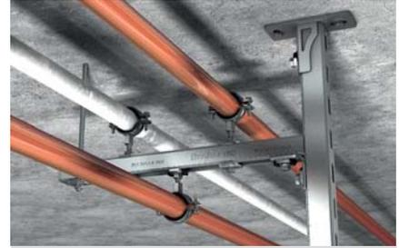
Cantilever construction with channel
