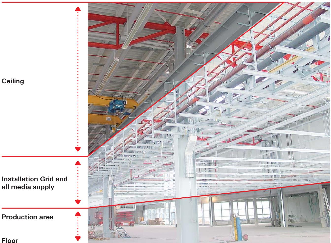
A separate level for the installation of media-supply equipment is constructed under the ceiling using a system of rails and special fixing elements from the fischer Installation Systems program. This Installation Grid can be specially adapted for any building.
